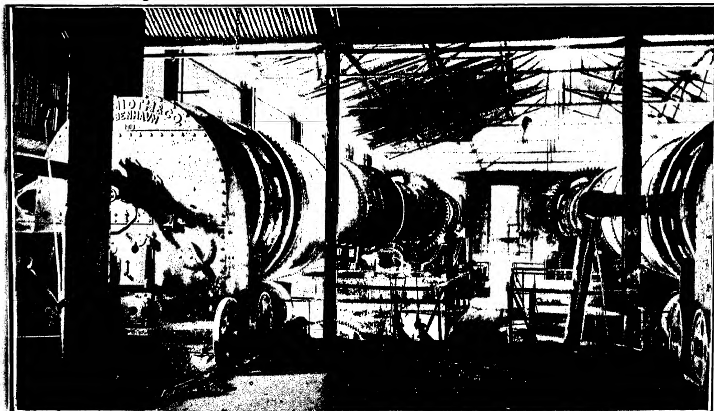
FIG. 2. ROTARY KILNS, BUNDI PORTLAND CEMENT WORKS, LAKHERI.
